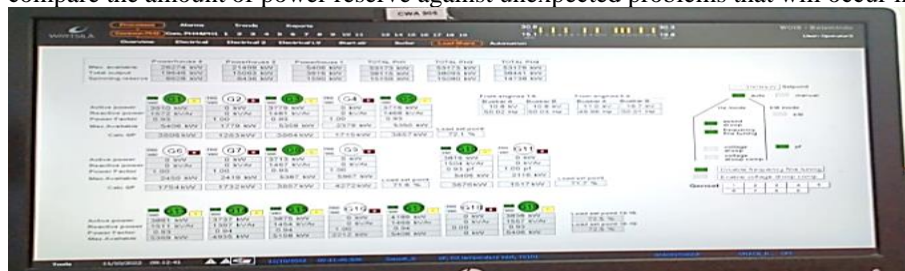
Figure 3.2. sWOIS screen display - Number of working generating machines
